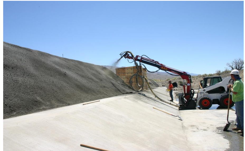
Shotcreting with KALMATRON® KF-A of irrigation system canals in Mojave Desert, California over of 100 °F without curing and isolation.
