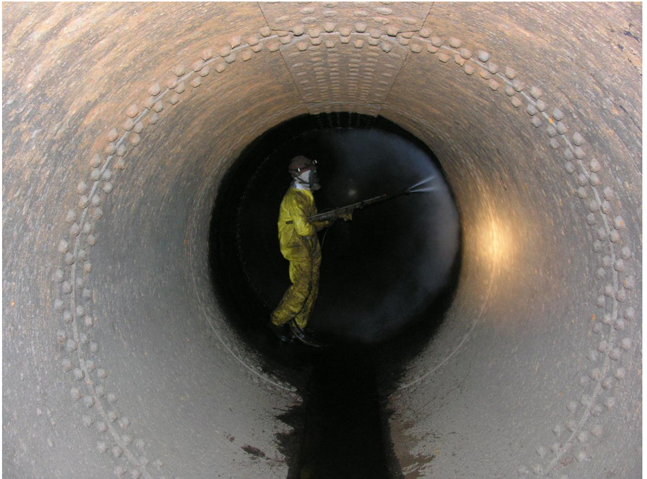
SHOTCRETING INSIDE PIPELINE
