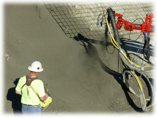
QUICK SAND STABILIZATION
